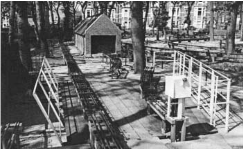
A photo of the main Traverser and Carriage Shed taken soon after completion
