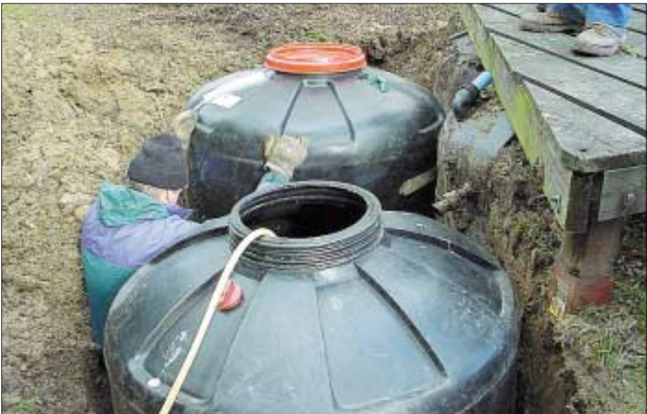
BOTTOM: Installing additional water storage at Canvey Railway & MEC. These barrels are used to transport orange juice from abroad and are subsequently available at a very favourable price. Nine drums are now in place; each has a capacity of 370 gallons and are used to collect rainwater from station buildings, etc.
